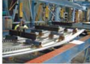
Formwork - Point Load
