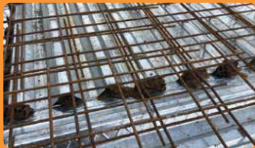
Sealing of opening & lapping
