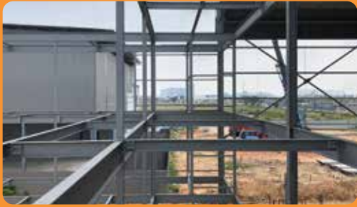
Installation of structure
