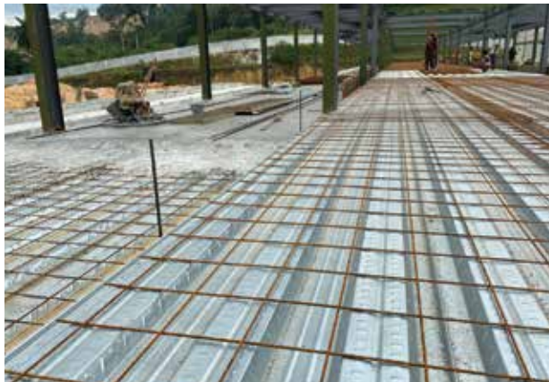
Continuous Span Installation
