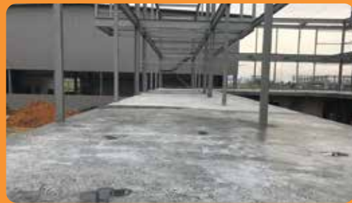
Concrete floor curing
