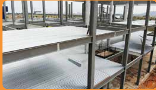
Laying of floor deck
