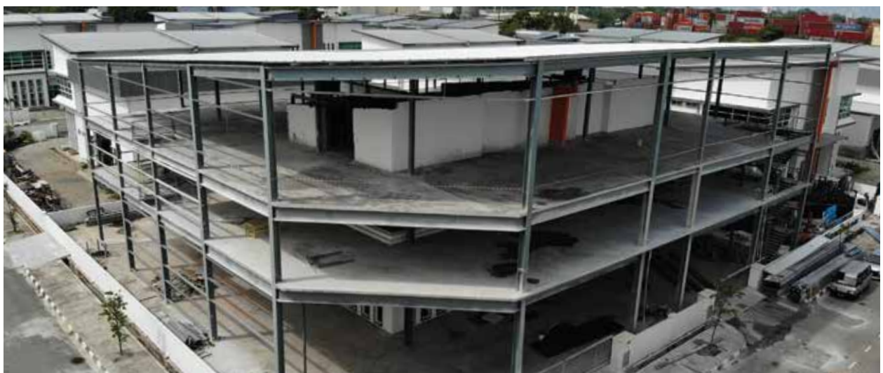
Warehouse Extension, Sg Lokan
