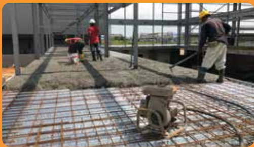
Concrete mixture levelling
