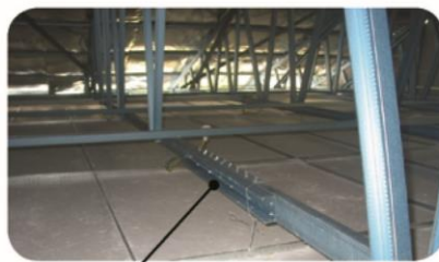
Bottom chord splice joint
